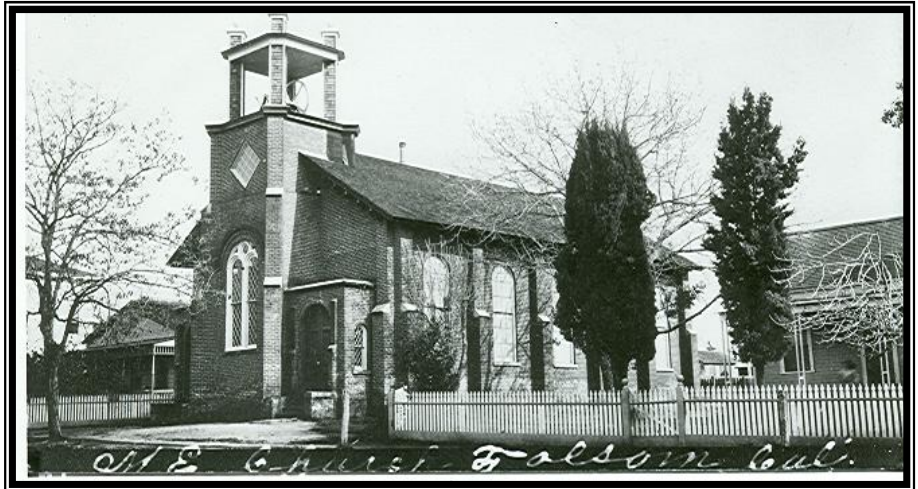
Built by Folsom Methodists 1860—Photo From Fall 1908
